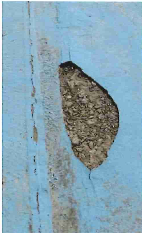
Delamination adjacent to construction joint
