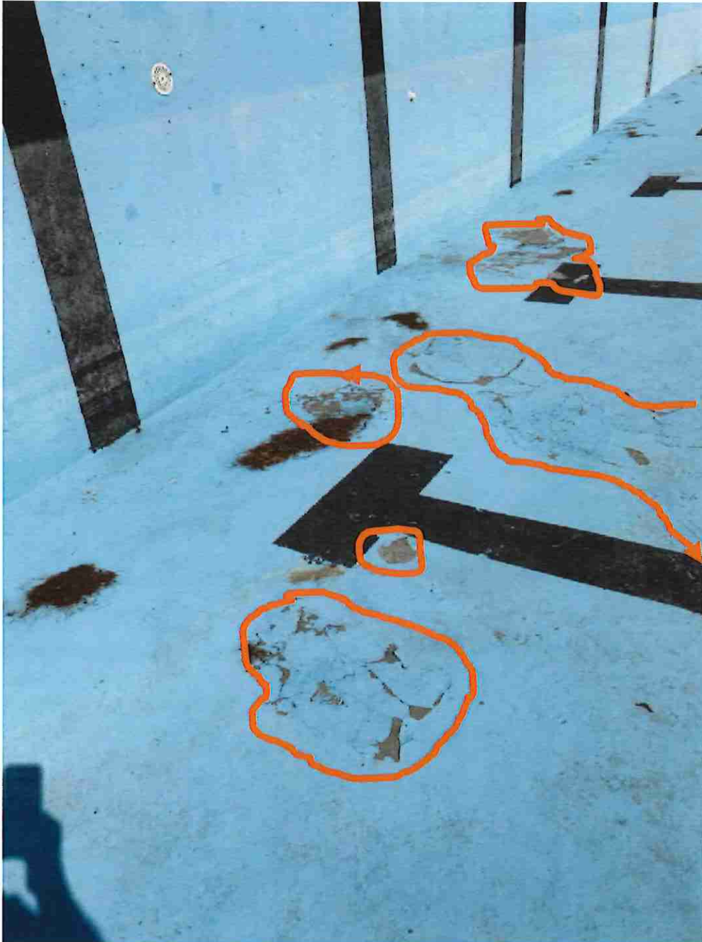
Broad areas of spalling and delamination
