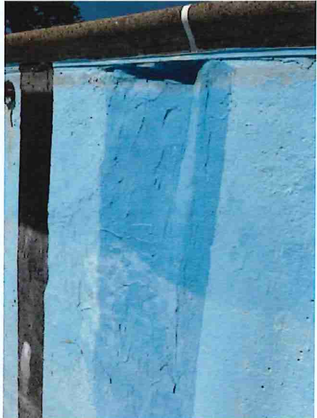
Significant spall of approximately 4-inches deep
