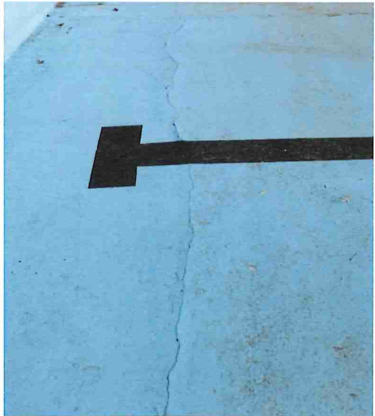
Typical crack in pool floor
