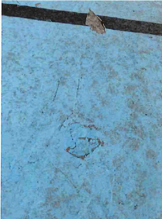
Multiple delaminations along the edge of crack
