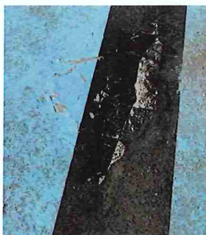
Previously repaired areas in pool floor with failure of repair materials
