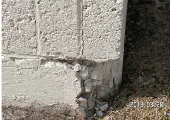
Figure 31 – Foundation spalling
