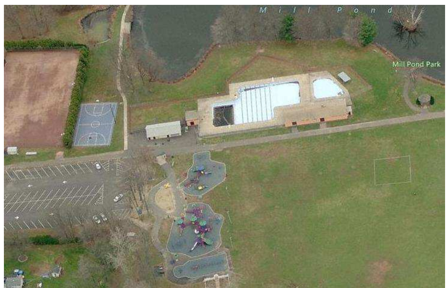
Figure 2 – Overview of Mill Pond Pool facility
